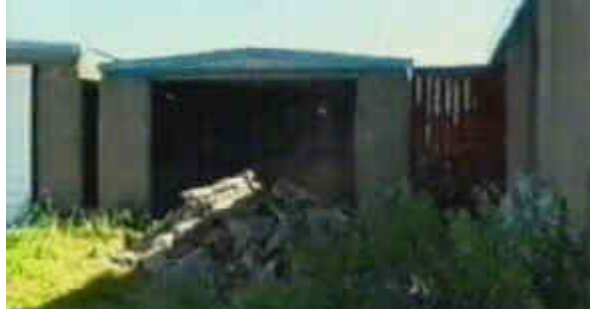
The Garage where the concrete block was found
