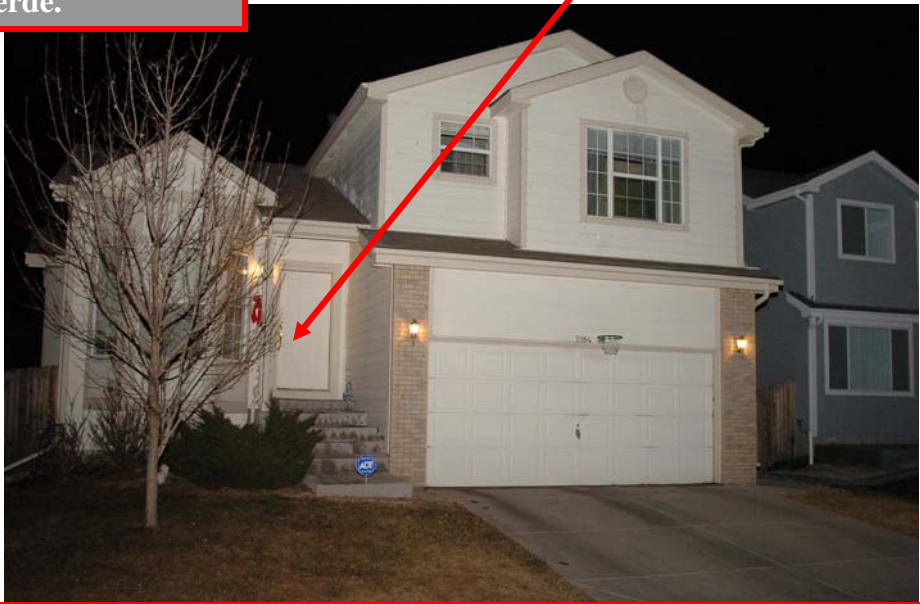
Photo looking East from Fontana Court at 5184 Fontana Court.
