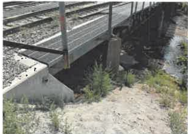
Figure 3. The opening to the area under the railroad bridge.
